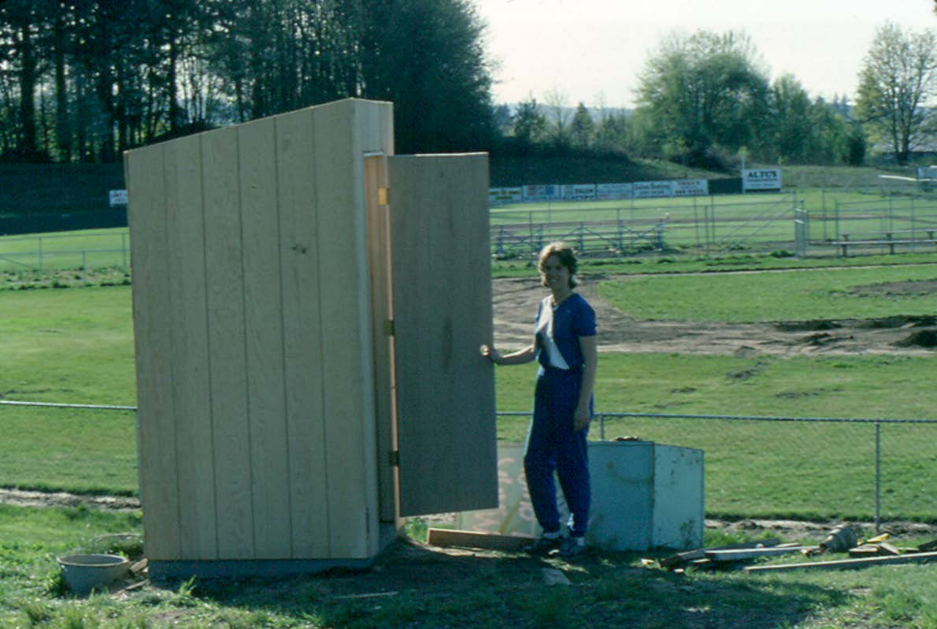
Bev Cox inspects the new pump house
